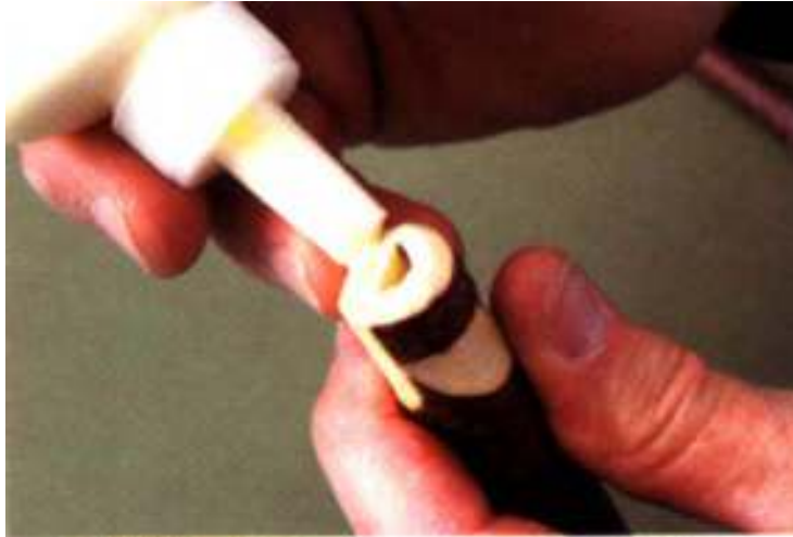
Figure A-11 Glue Cracks
