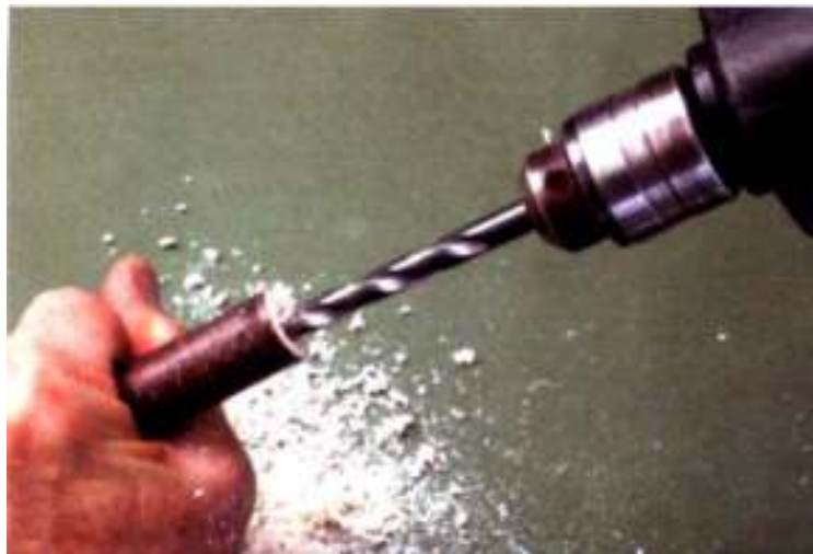
Figure A-1 Drill a Hole
